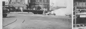
9 a.m. Steel cable wrapped around second story of old Marine Annex Building is pulled taut in readiness to raise the structure simply and quickly. 9 a.m. Cable di staal bora rond di segundo piso di Marine Annex Building biewu ta wordo pretu pa hala e bora basha abao simple y biera.
